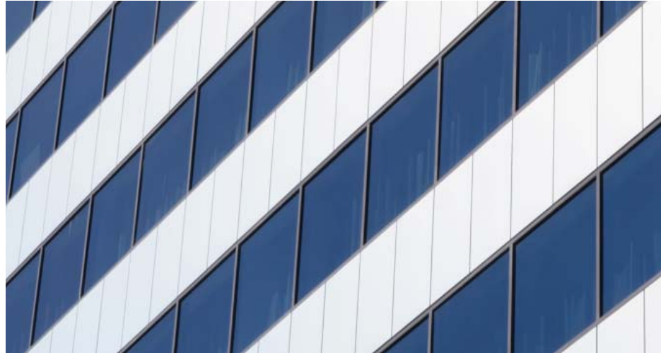
Image 25: Spandrels interrupting a reflective facade
