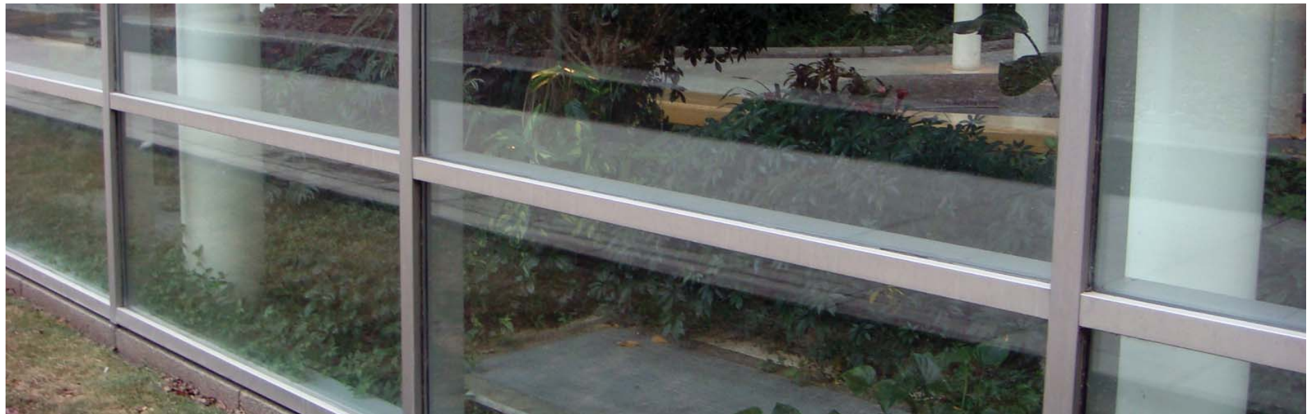
Image 35: Lobby landscaping visible from the exterior
