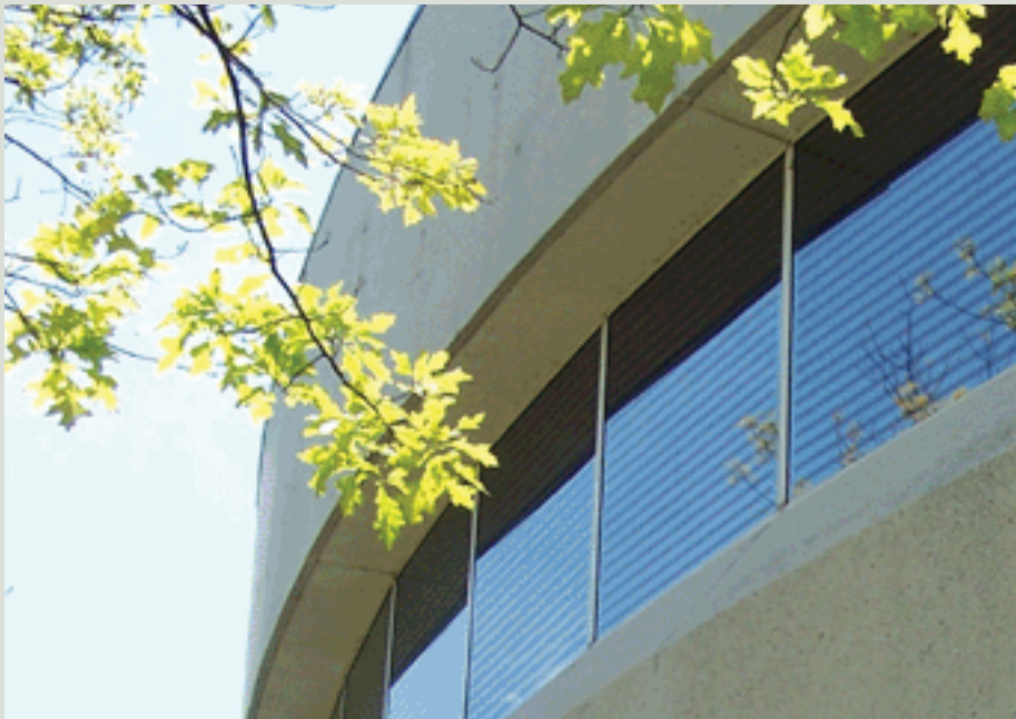
Image 19: A window film applied to the solarium entrance of a town building in Markham, Ontario to prevent bird-window collisions
