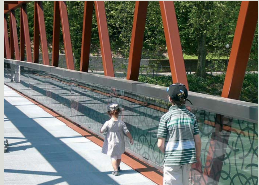
Image 20: Translucent visual marker treatment on a bridge guardrail
