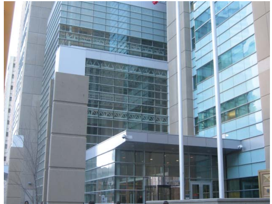
Image 22: The use of both transparent and opaque building surface materials combined with dense mullions.
